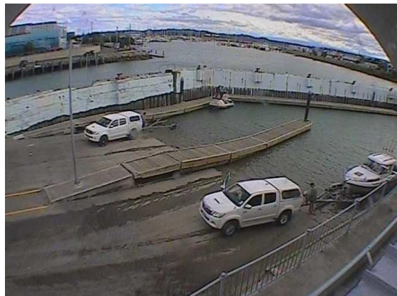
Figure 10: Napier Sailing Club Boat Ramp wind break screens.
