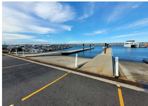
Figure 6: Augusta boat ramp.
